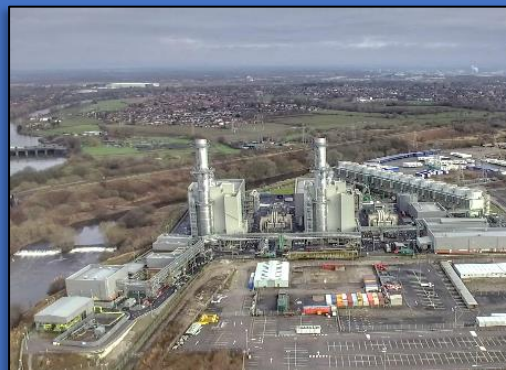
Large gas plant
